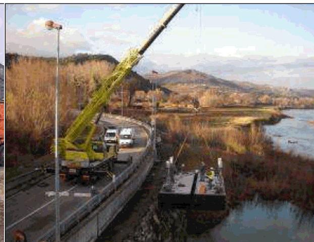
Figure 79 –Atelier de forage
